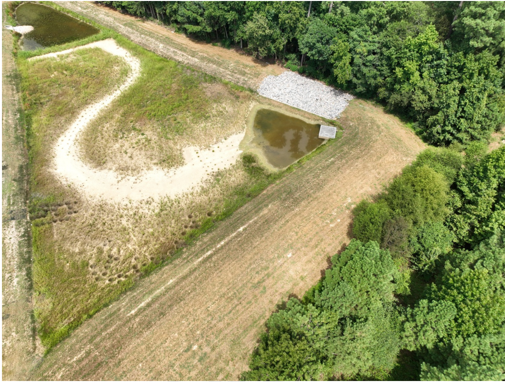
Fig. 2 — Stormwater control measure aerial view: forebay with sediment accumulation, permanent pool, outlet structure and rip-rap emergency spillway.
