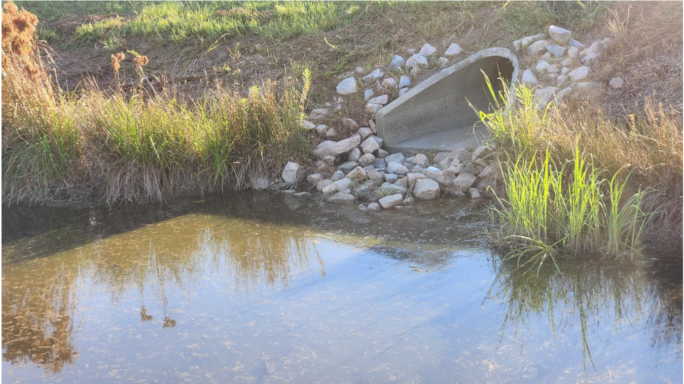
Fig. 1 — Stormwater control measure outfall. Reinforced concrete pipe with riprap stone apron discharging to the permitted pond. Riprap coverage extends approximately eight feet from pipe outlet; grass cover along bank established, no debris blocking outlet.
