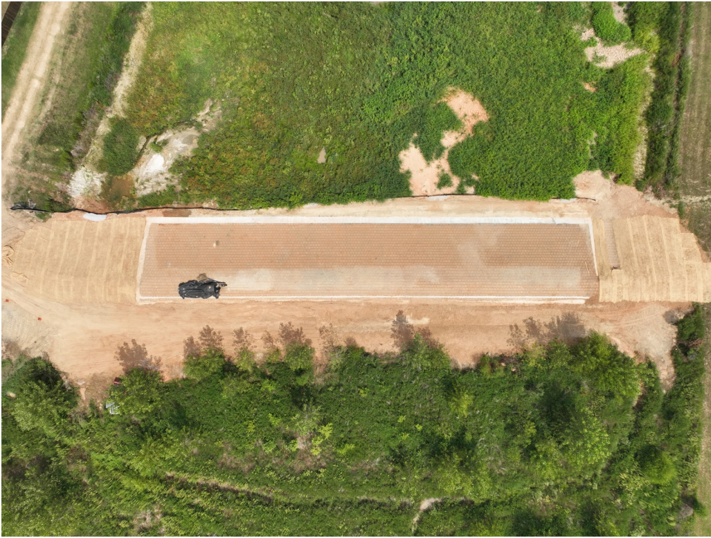
Fig. 8 — Maintained path; graded running surface and defined shoulders.
