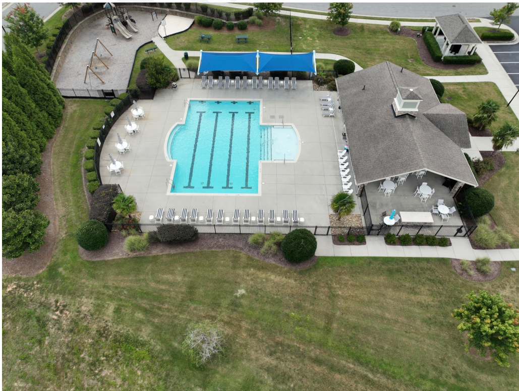
Fig. 3 — Amenity center and pool deck on the date of flight. Roof, shade structures, deck, perimeter fencing and furniture in a single orienting frame.
