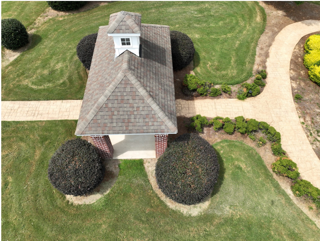
Fig. 5 — Picnic pavilion, photographed from directly overhead; roof surface, walkway and surrounding beds.
