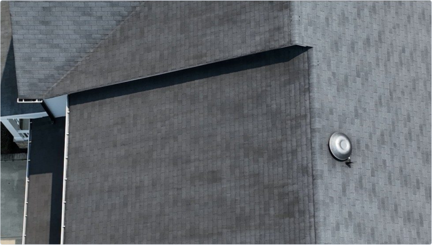
Fig. 7 — Perimeter and vent cluster. Vents seated; no displacement observed.
