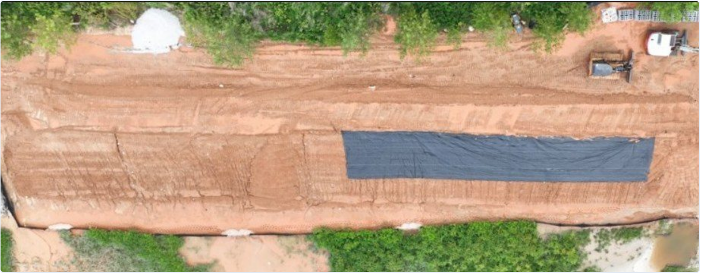
Fig. 2 — Plan (near-nadir) view. Graded corridor and culvert crossing, photographed vertically so the same frame can be repeated on every visit.
