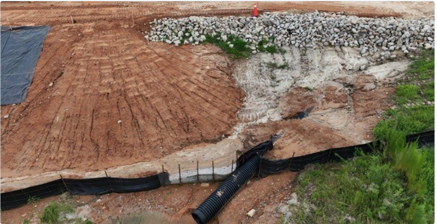
Fig. 5 — Erosion-control detail. Rip-rap apron and outlet protection as installed, at low altitude.
